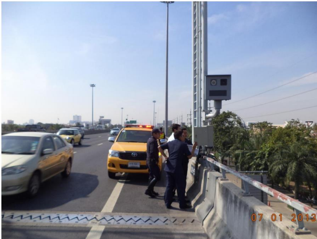
Figure 3.4 Speed Enforcement Camera at KM 12+500A on Chalongrat Expressway, Northbound
