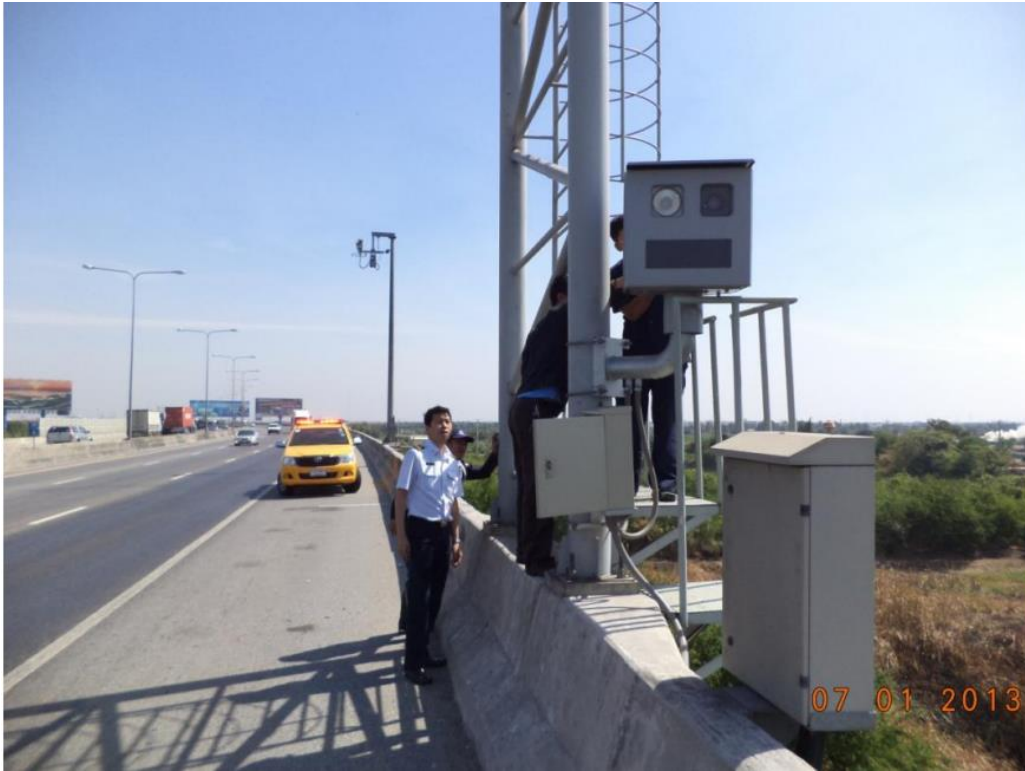
Figure 3.15 Backup Site at KM 8+000B on Kanchanapisek Expressway, Eastbound
