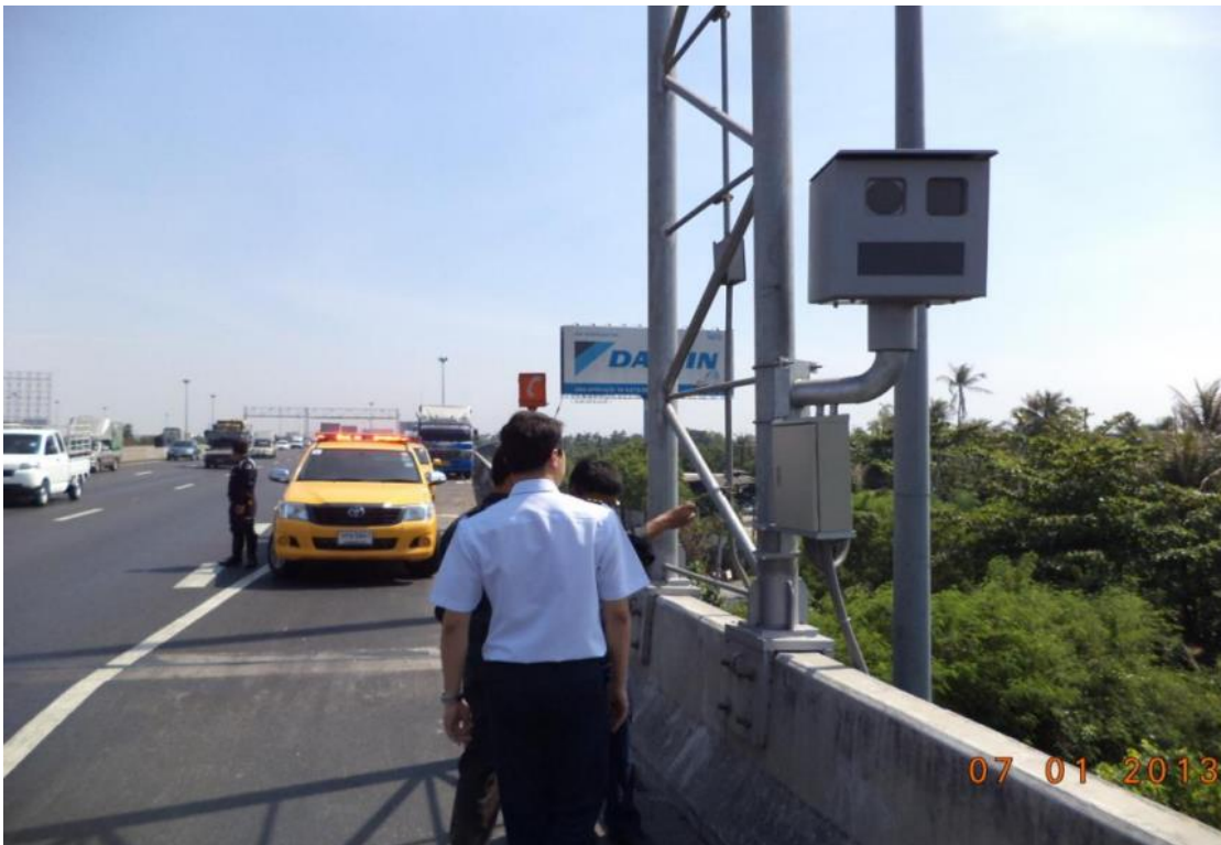
Figure 3.16 Backup Site at KM 17+800A on Kanchanapisek Expressway, Westbound
