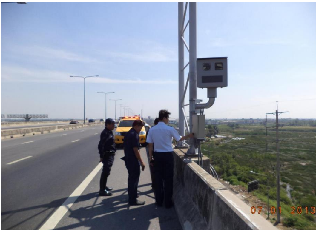
Figure 3.18 Backup Site at KM 30+700 (Inbound) on Burapha Withi Expressway, Westbound
