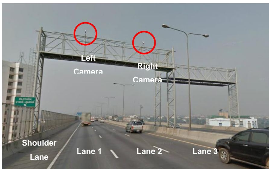
Figure 3.21 Appearance of image processing cameras and lane configuration on the Kanchanapisek expressway (station KM 8+000A)
