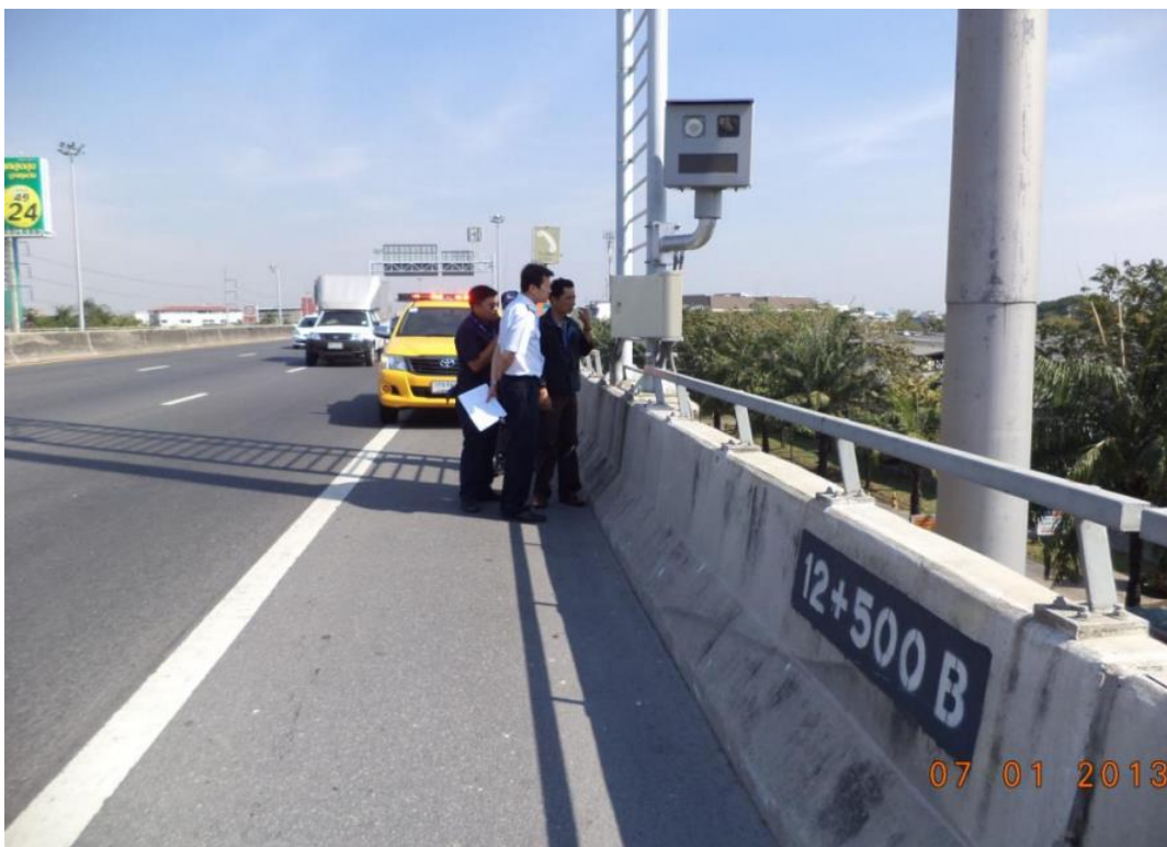
Figure 3.5 Speed Enforcement Camera at KM 12+500B on Chalongrat Expressway, Southbound
