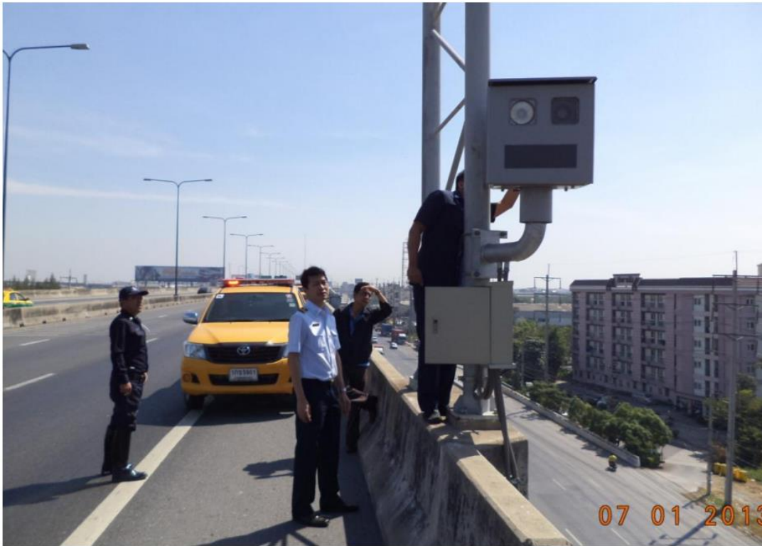
Figure 3.11 Speed Enforcement Camera at KM 14+050 (Inbound) on Burapha Withi Expressway, Westbound
