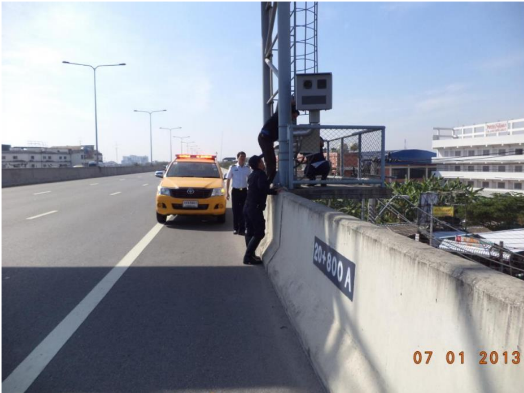
Figure 3.13 Backup Site at KM 20+800A on Chalongrat Expressway, Northbound
