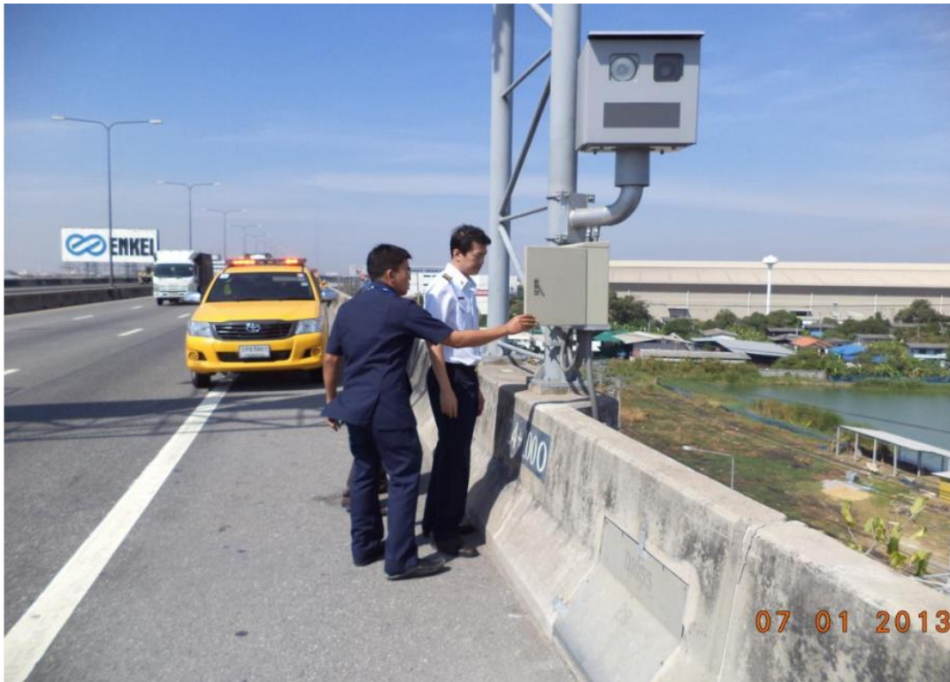
Figure 3.17 Backup Site at KM 14+000 (Outbound) on Burapha Withi Expressway, Eastbound
