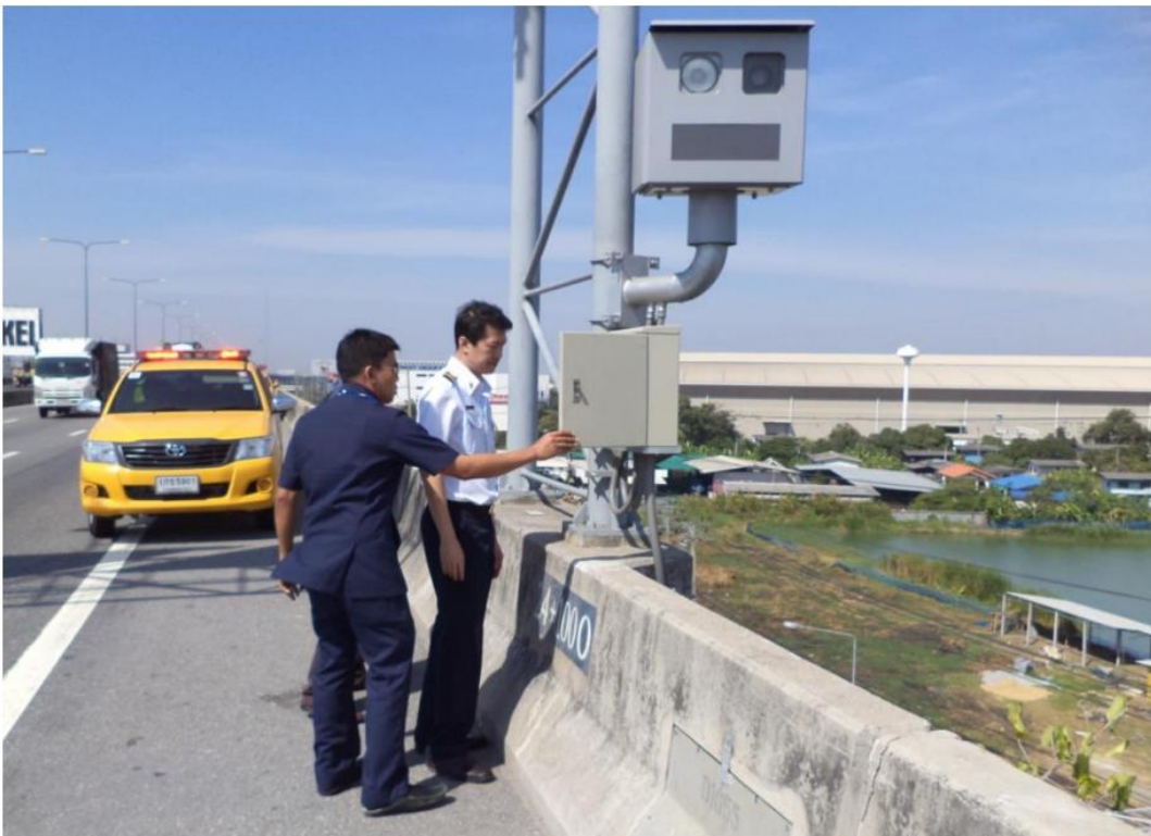
Figure 3.12 Speed Enforcement Camera at KM 24+100 (Outbound) on Burapha Withi Expressway, Eastbound
